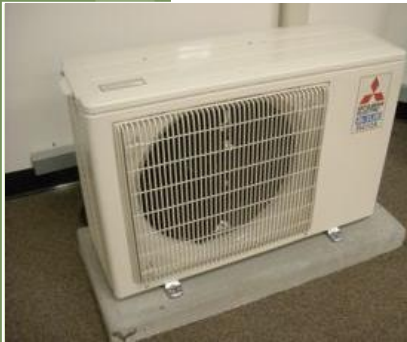
Ductless heat pump condensing unit
