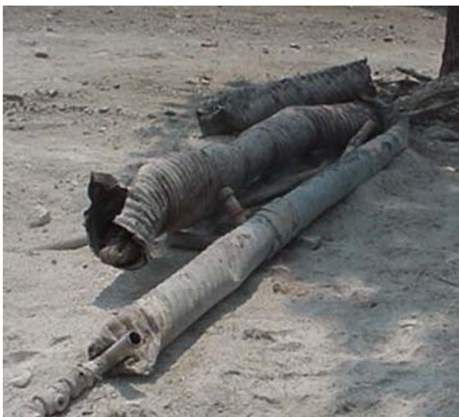
Figure 9: Asbestos-Containing Steam Pipe
