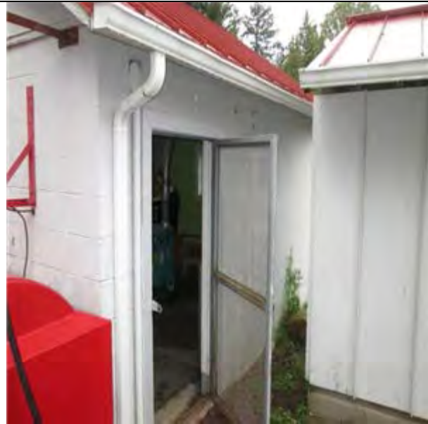
B2039 Other Doors & Entrances.1:- View of mesh door.
