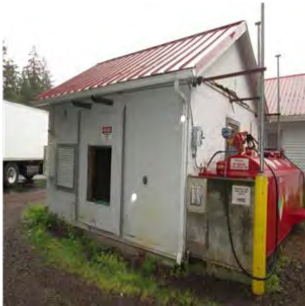
B3011 Roof Finishes.1:- A view of the corrugated roof finish.
