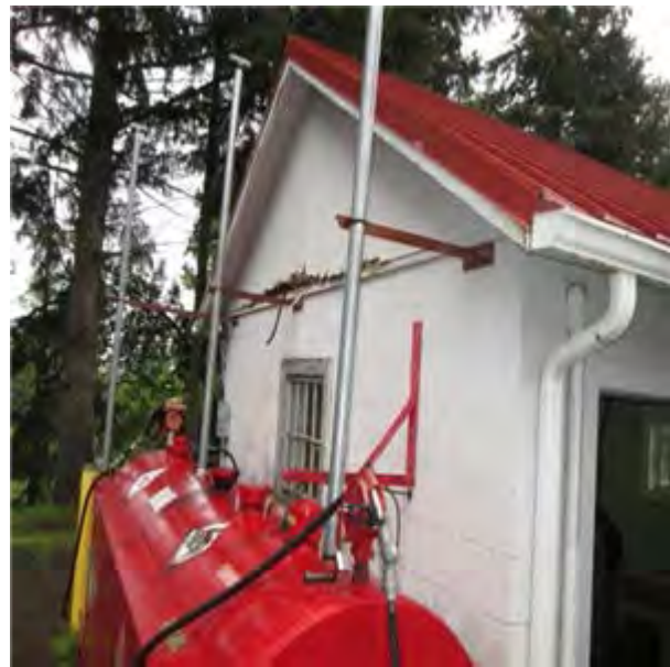
B3016 Gutters and Downspouts.1:- View of the gutter and downspout.
