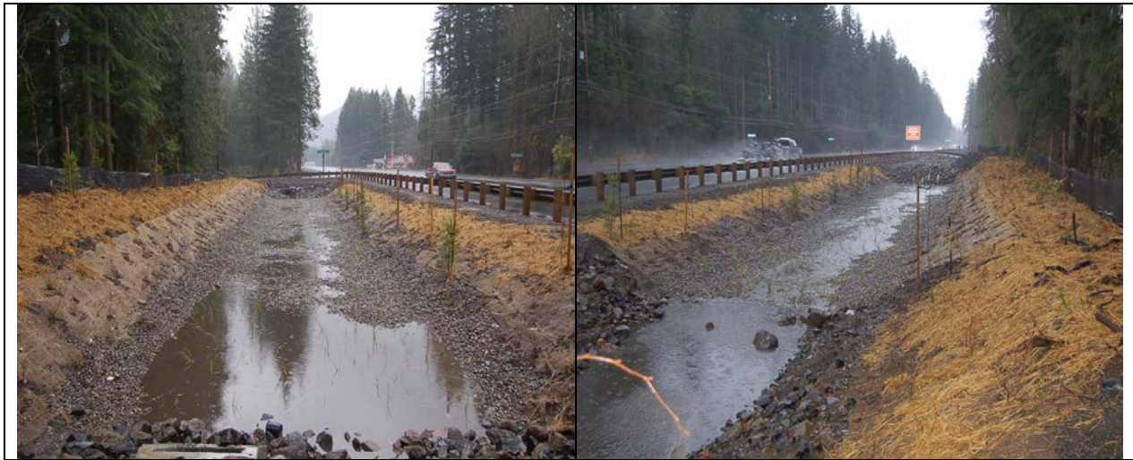
Figure 1 Extended detention dry pond
