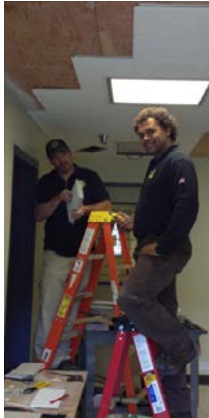
Dennis Padilla (left) and Steve Babcock install ceiling tiles.
