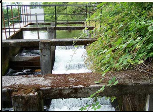
Lower Bennett fish passage facility
