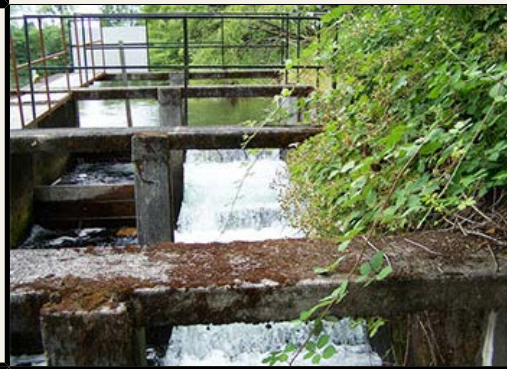
Lower Bennett fish passage facility
