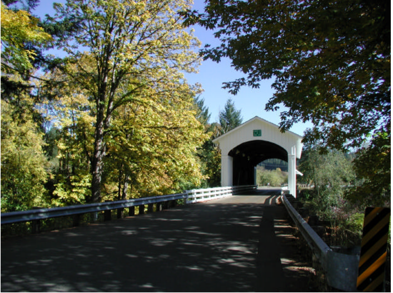
Earnest Covered Bridge
