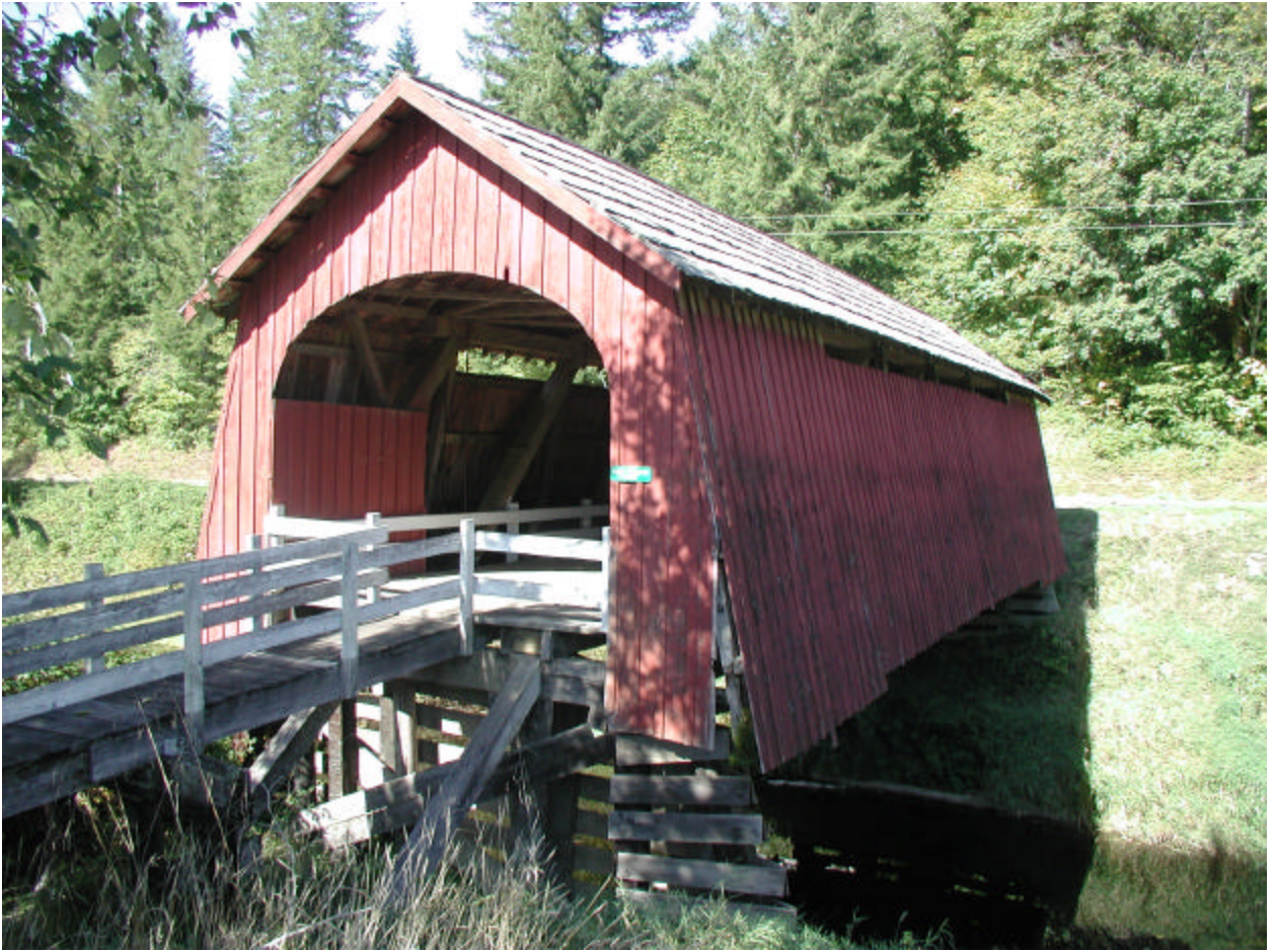
Fisher School Covered Bridge
