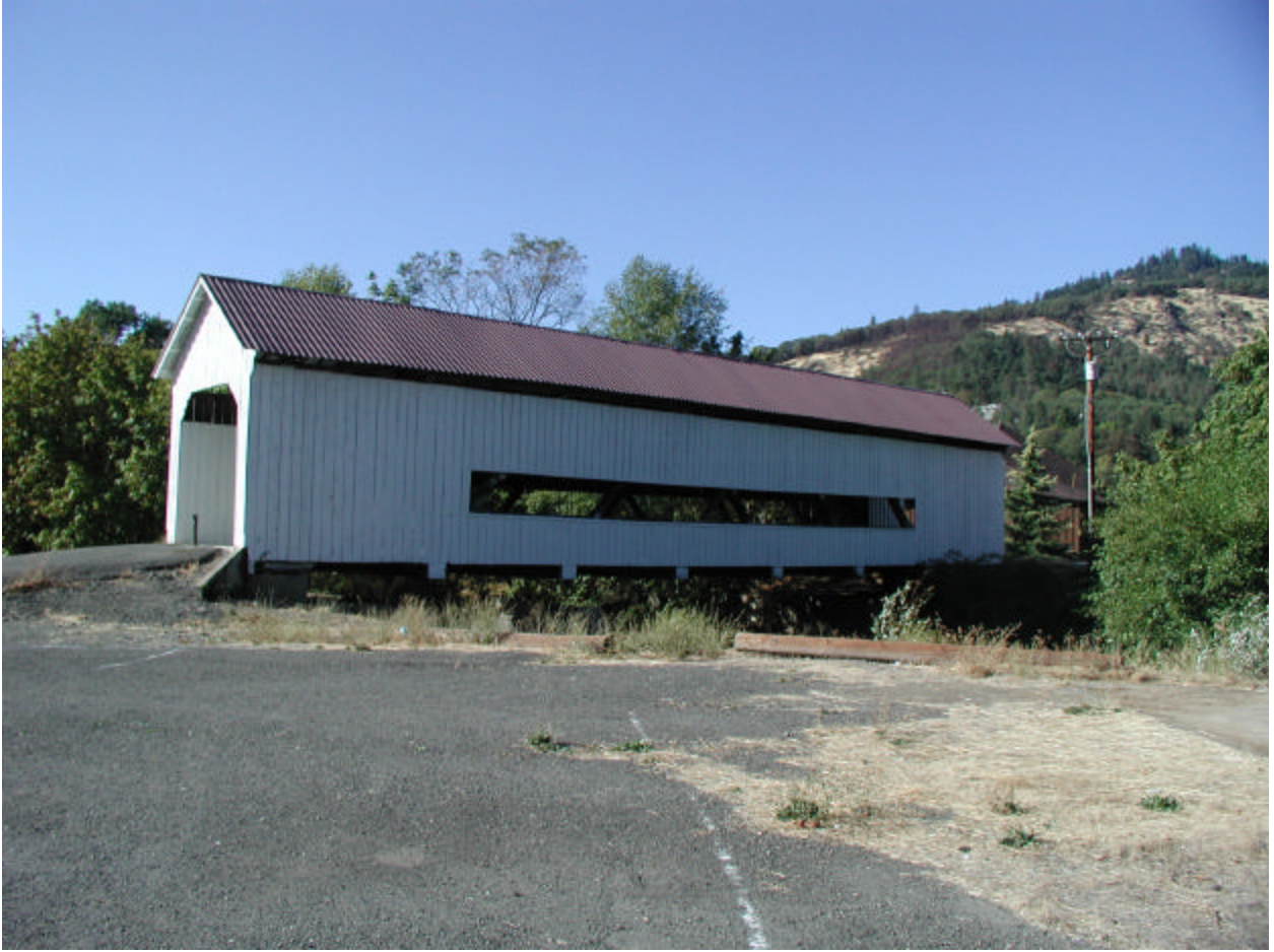
Horse Creek Covered Bridge
