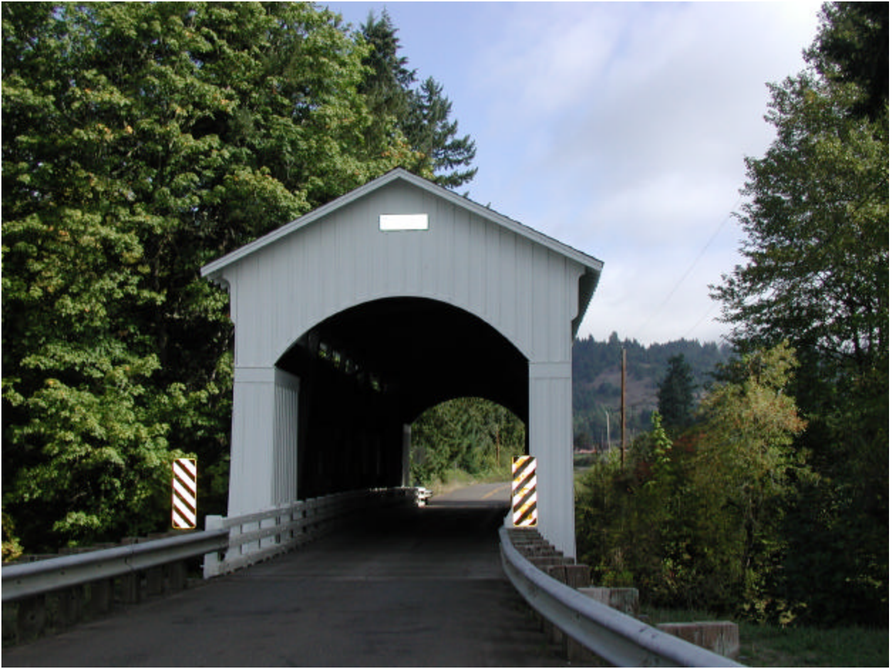
Mosby Creek Covered Bridge
