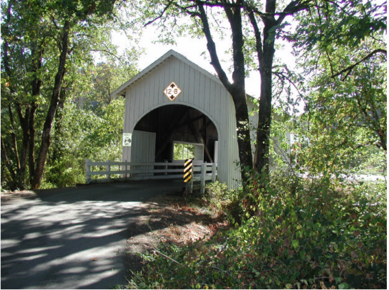
Neal Lane Covered Bridge
