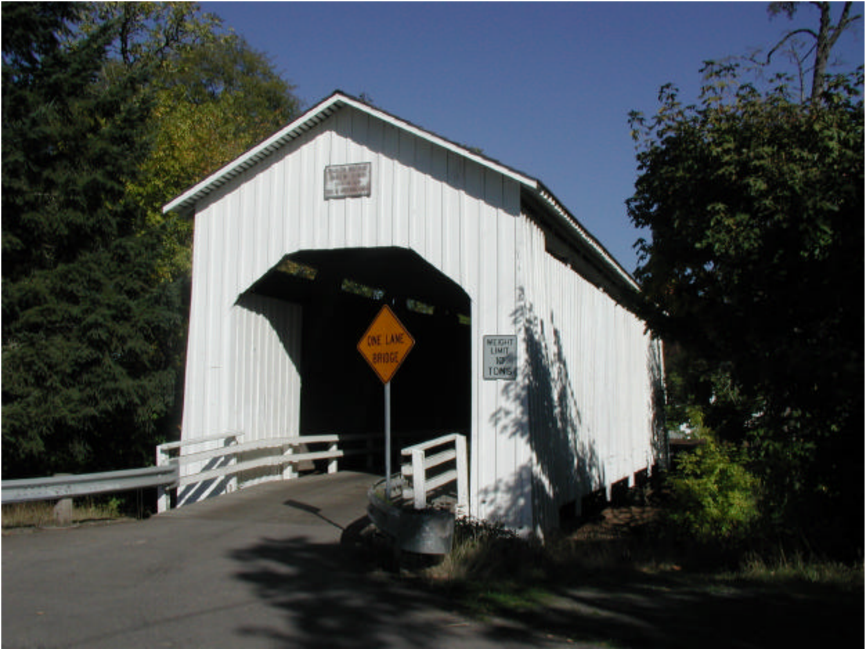
Parvin Covered Bridge
