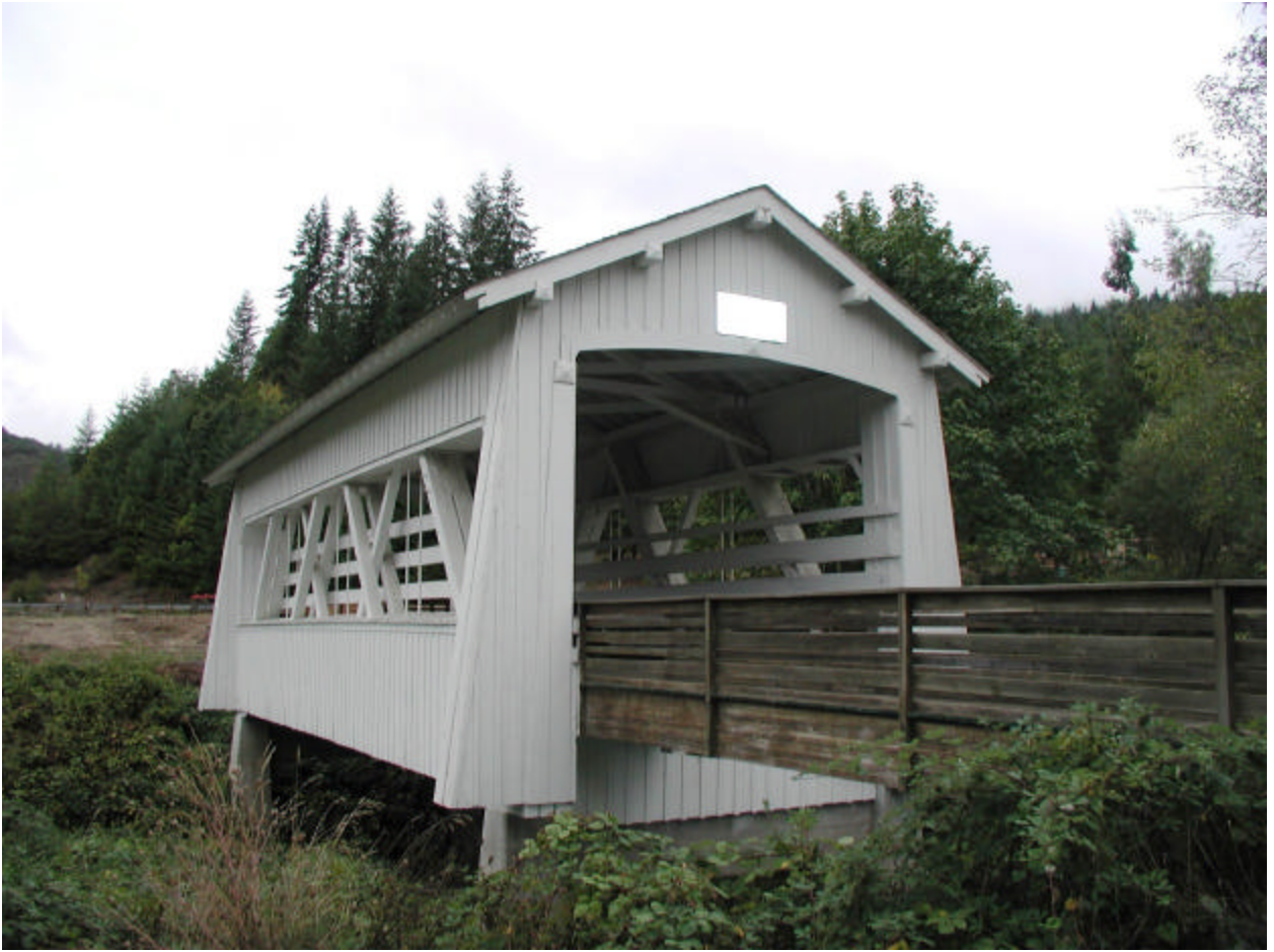
Sandy Creek Covered Bridge
